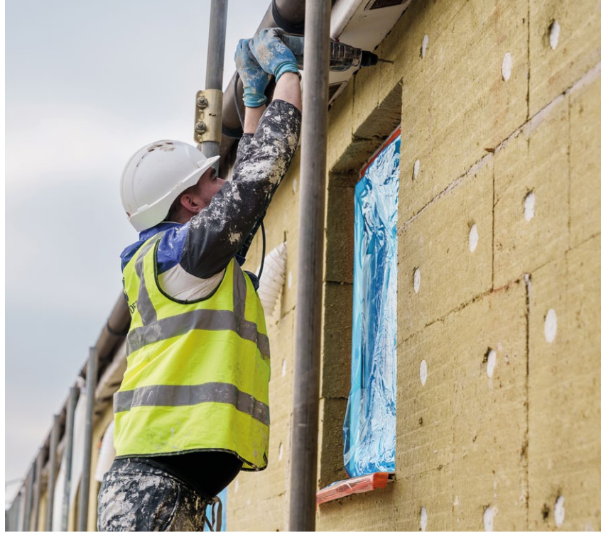
Fitting external wall insulation.
