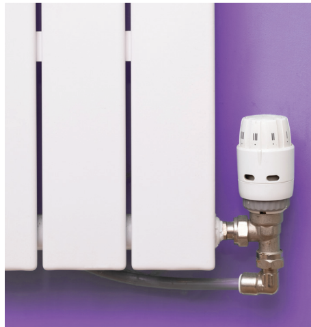
Thermostatic radiator valve (TRV). ↘
